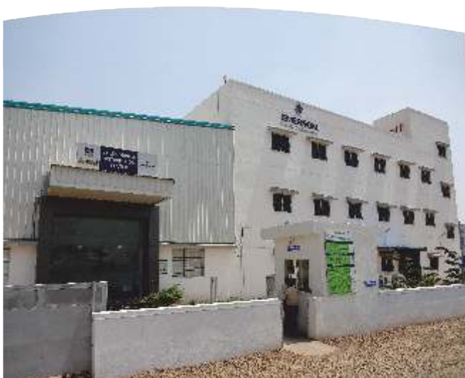
Cold Chain & Distribution Center
