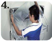
4.Place the closed type cleaning cover on C shaped support bracket, insert those two small transparent films on both side in the back of the air conditioner.
