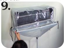
9.Finally pull up rope stoppers around the four corners to the same level to finish the installation.
