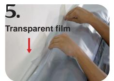
5.Insert the big size of transparent film in the back of the air conditioner and tighten the cleaning cover by adjust the rope stopper.
