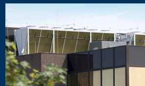
Grass Merkur Data Centre Hannover, Germany
